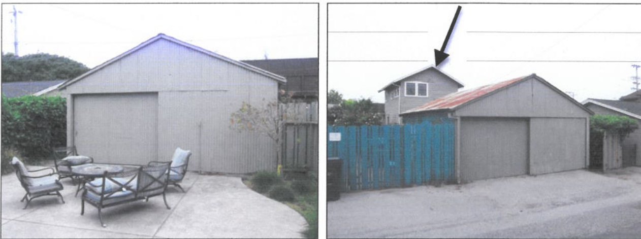
Figures 3 and 4. Left image shows the west elevation of the garage taken from the backyard. Right image shows the garage's east elevation facing the Grand Avenue alley. The main house's second story addition appears behind the garage (arrow).
